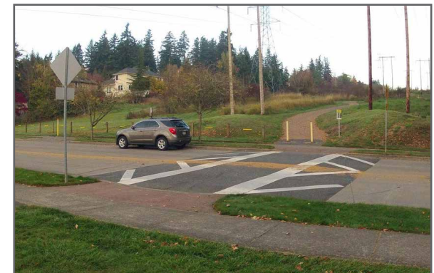
Raised crosswalks double as vertical traffic calming elements
