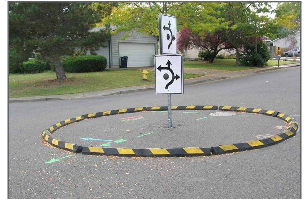
Mini traffic circles can be created using temporary materials, such as rubber curbs
