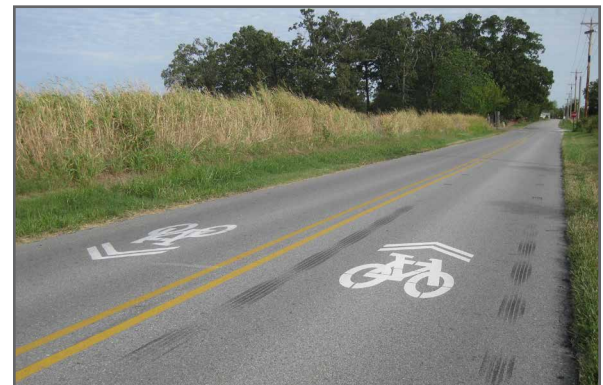
Shared lane markings in the middle of the travel path increases the longevity of the markings
