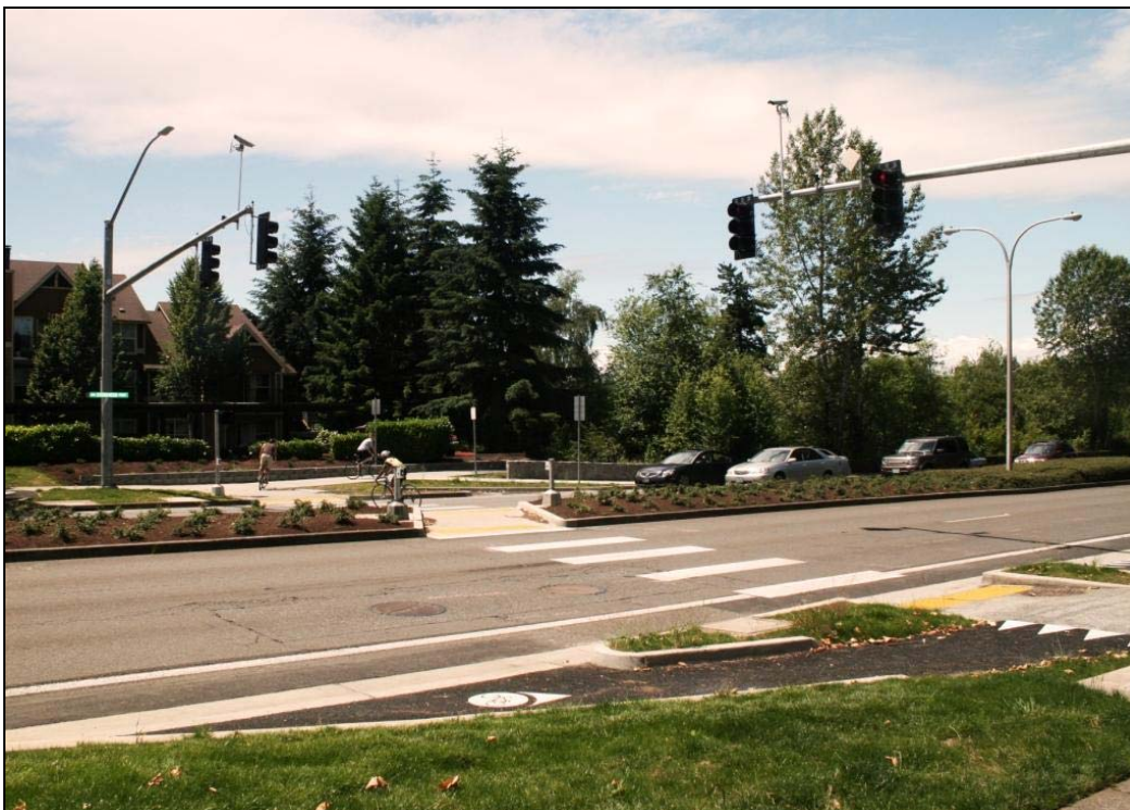
Mid-block crossings like this example (Rock Creek Trail at NW Evergreen Parkway) can help neighborhood bikeways cross large arterial roads.
