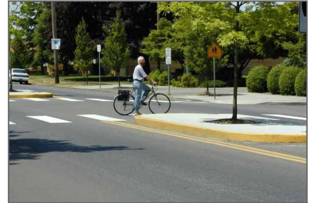
Median refuge islands enhance the safety and comfort of midblock crossing locations.
