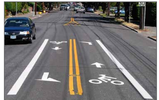
Bike left turn lanes help bicyclists conveniently navigate jogs in the Neighborhood Bikeway route
