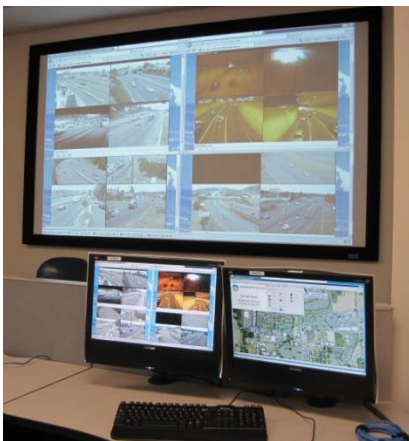
Video wall and workstation at the Traffic Operations Center
