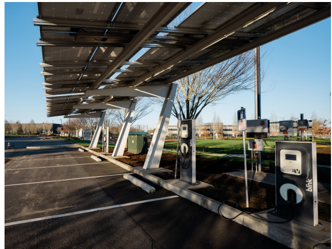
FIGURE 16. ELECTRIC VEHICLE CHARGING STATION
