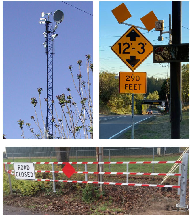
FIGURE 14. (TOP LEFT) ROADWAY WEATHER INFORMATION SYSTEM, (TOP RIGHT) OVERHEIGHT WARNING FLASHES WHEN APPROACHING VEHICLE EXCEEDS HEIGHT LIMIT FOR UNDERPASS, (BOTTOM) GATE AT FERN HILL ROAD CAN BE CLOSED WHEN ROADWAY FLOODS
