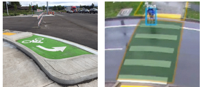
FIGURE 13. PEDESTRIAN/BICYCLE DETECTION USING EMBEDDED SENSORS, OR THERMAL/VIDEO TECHNOLOGY TO IMPROVE SAFETY
