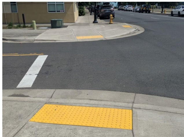
CURB RAMP IMPROVEMENTS
