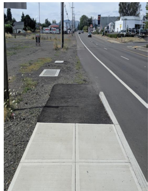
Sidewalk abruptly ends and turns to gravel along roadway at Adair/Baseline and 10th Avenue
