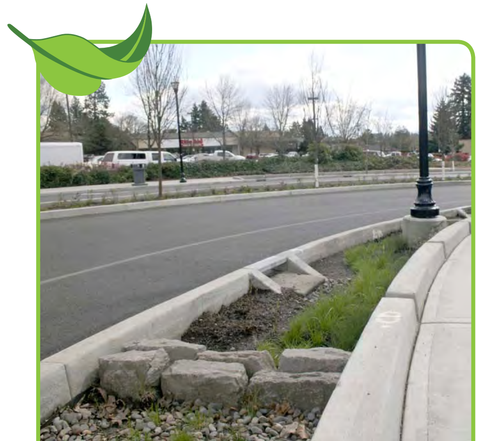
The City of Tigard incorporated a vegetated drainage swale in the reconstruction of a portion of Main Street in 2011.
