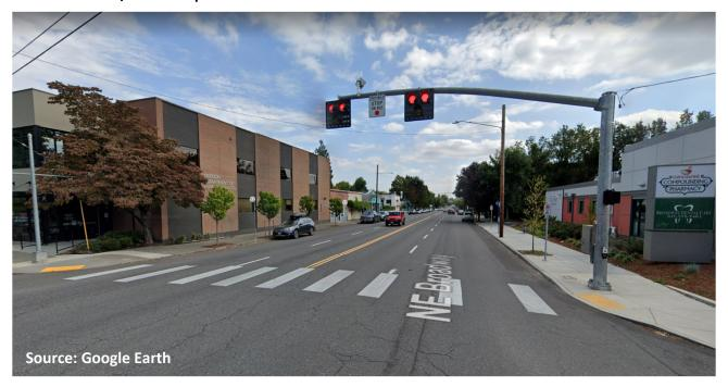
The example shown in Exhibit 3 is a typical application of a HAWK / PHB signal. This HAWK / PHB example is located on a four-lane roadway with two travel lanes in both directions. The HAWK / PHB signal is mounted on a mast arm along with crosswalk signage.
