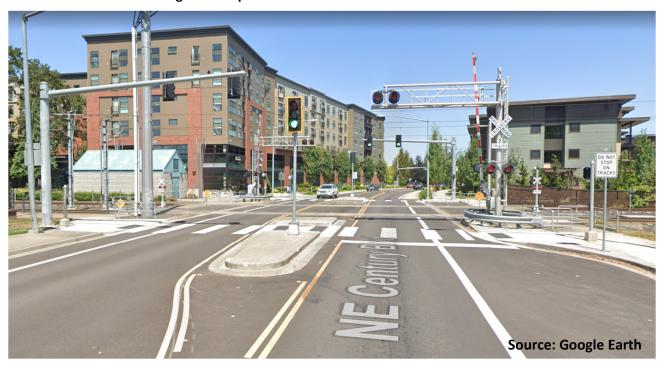
The example shown in Exhibit 4 is located just east of the Orenco/NW 231<sup>st</sup> Avenue MAX station and programmed to be coordinated with the railroad signals and infrastructure.
