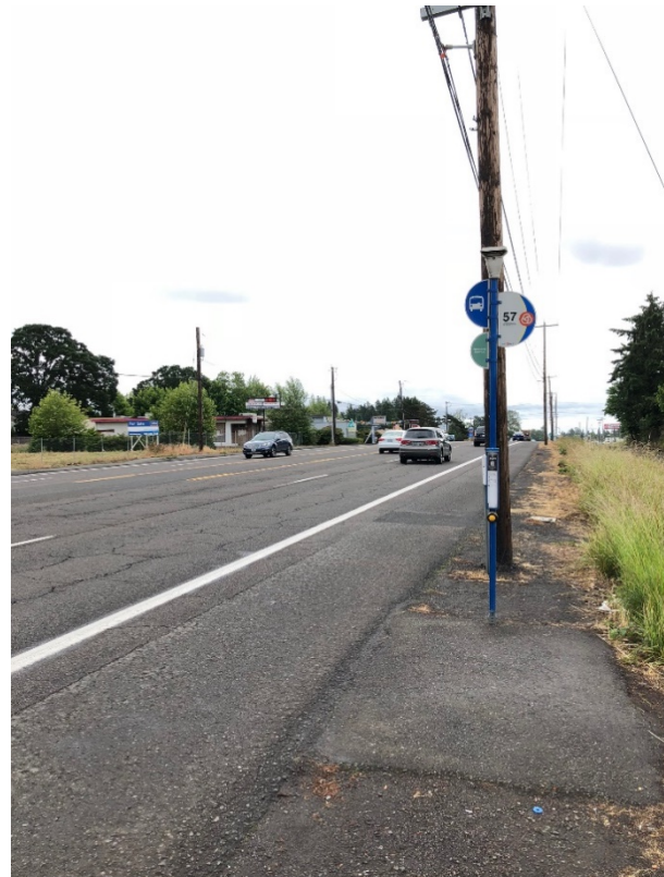
The eastbound bus stop at 174 th Avenue and TV Highway lacks sidewalks and striped crossings to safely and effectively access transit.
