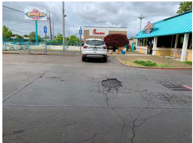
At southeast corner of site looking west. Pavement damage observed in form of pop-outs, alligator cracking, and depressions.
