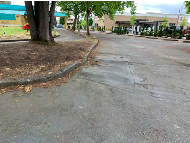
At western side of site looking south. Large roots of mature tree have caused damage of pavement in form of heave and cracking. It appears repairs to the pavement in this area have been made in the past. Also, longitudinal crack in pavement above existing utility along access drive.
