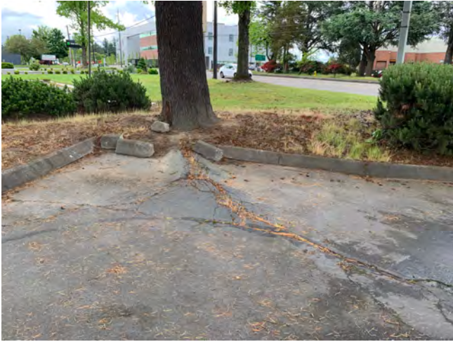
At southeast corner of site looking southeast: large roots of mature tree causing extensive damage of pavement in form of heave and cracking.
