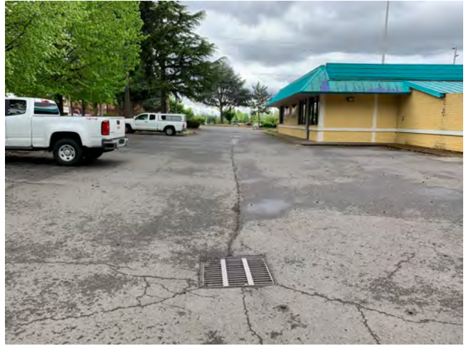
Near boring B-4 on east side of site looking south. Crack in pavement directly above existing utility line and emanating from hard corners of drainage grate.
