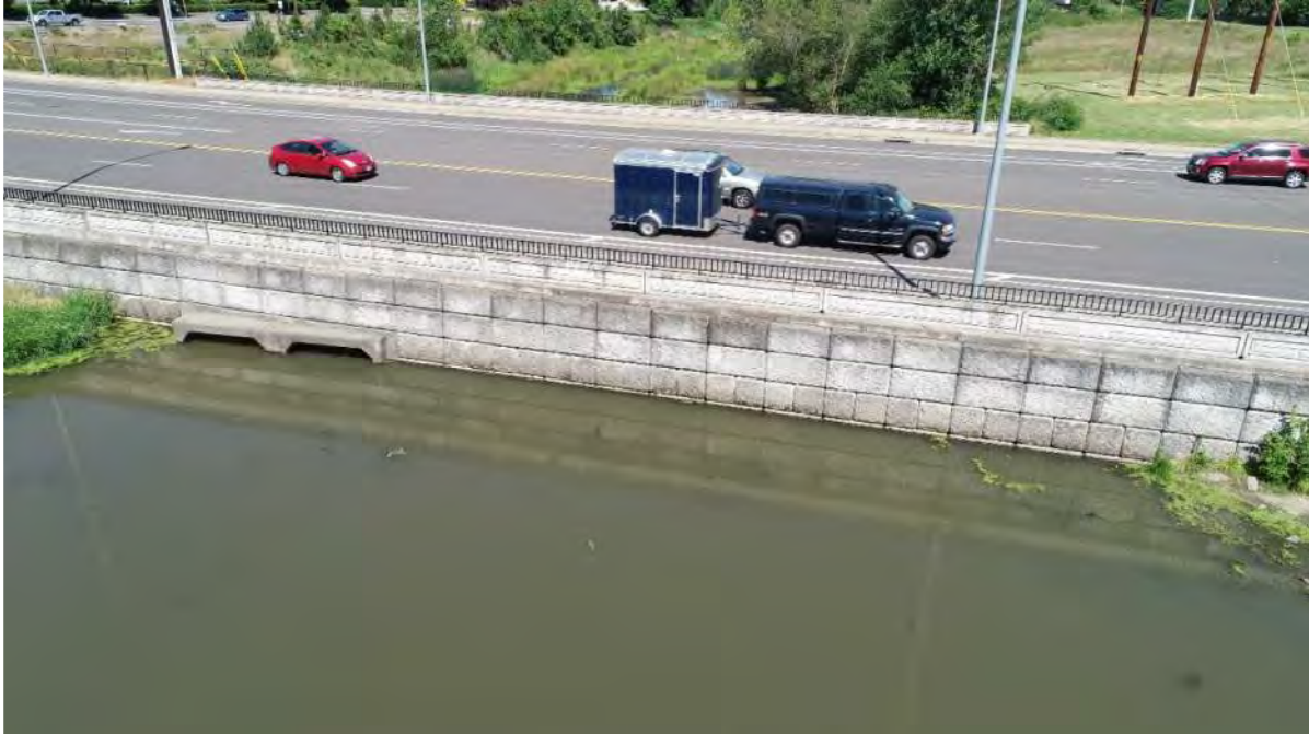
Downstream Side of Box Culvert Under NW 185 th Ave
