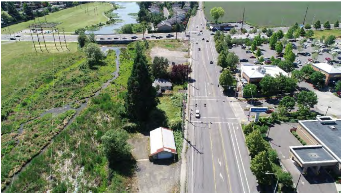
Overall Downstream System
