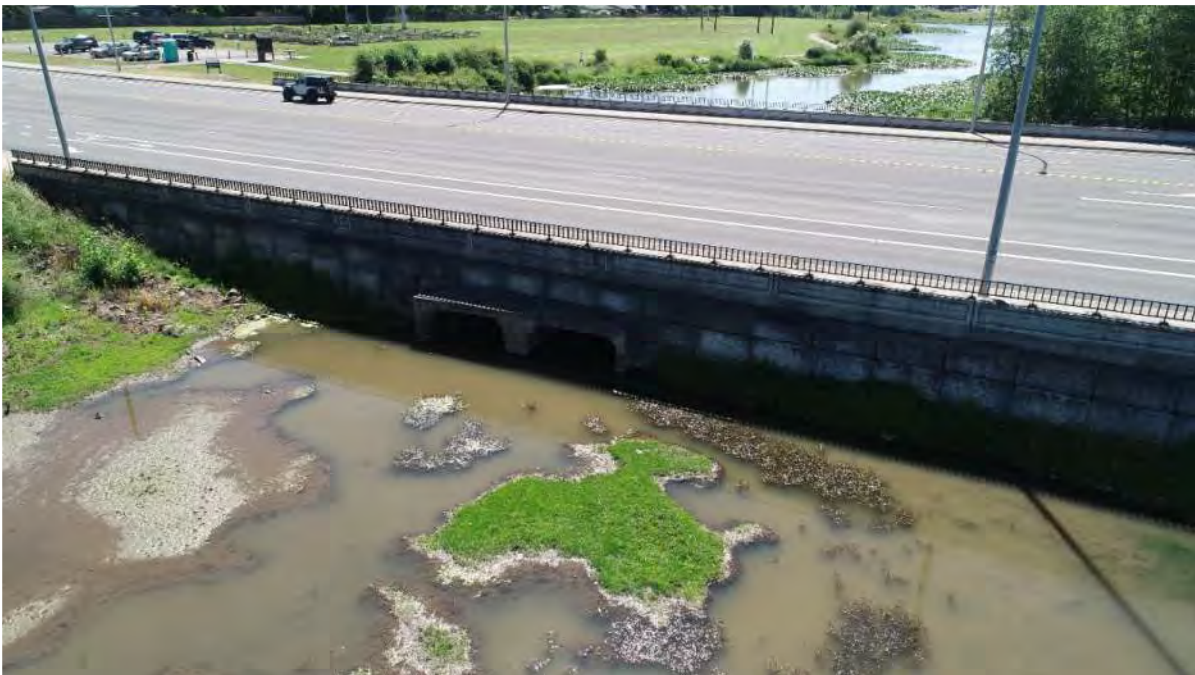
Upstream Side of Box Culvert Under NW 185 th Ave
