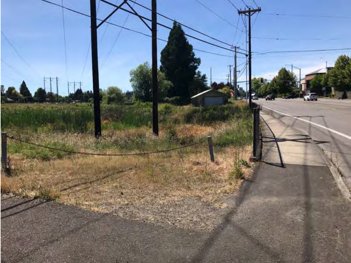
Downstream Discharge Area
